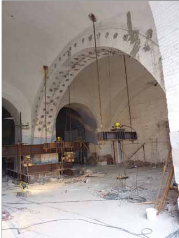
Figure 4 – Static test of Arch No.1 (Fig.1): application of the pull-down loads.
